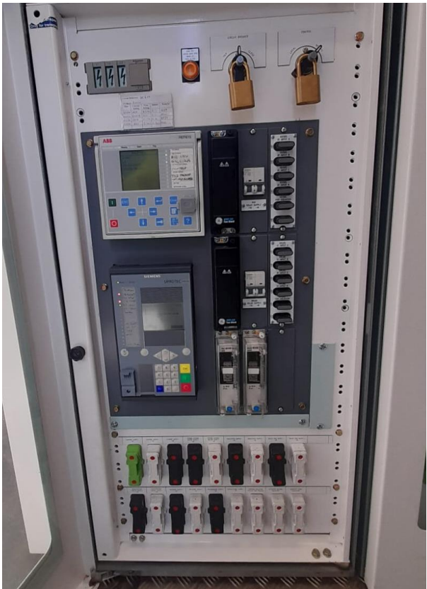
Figure 103: DER-4 PV – Protection Panel
