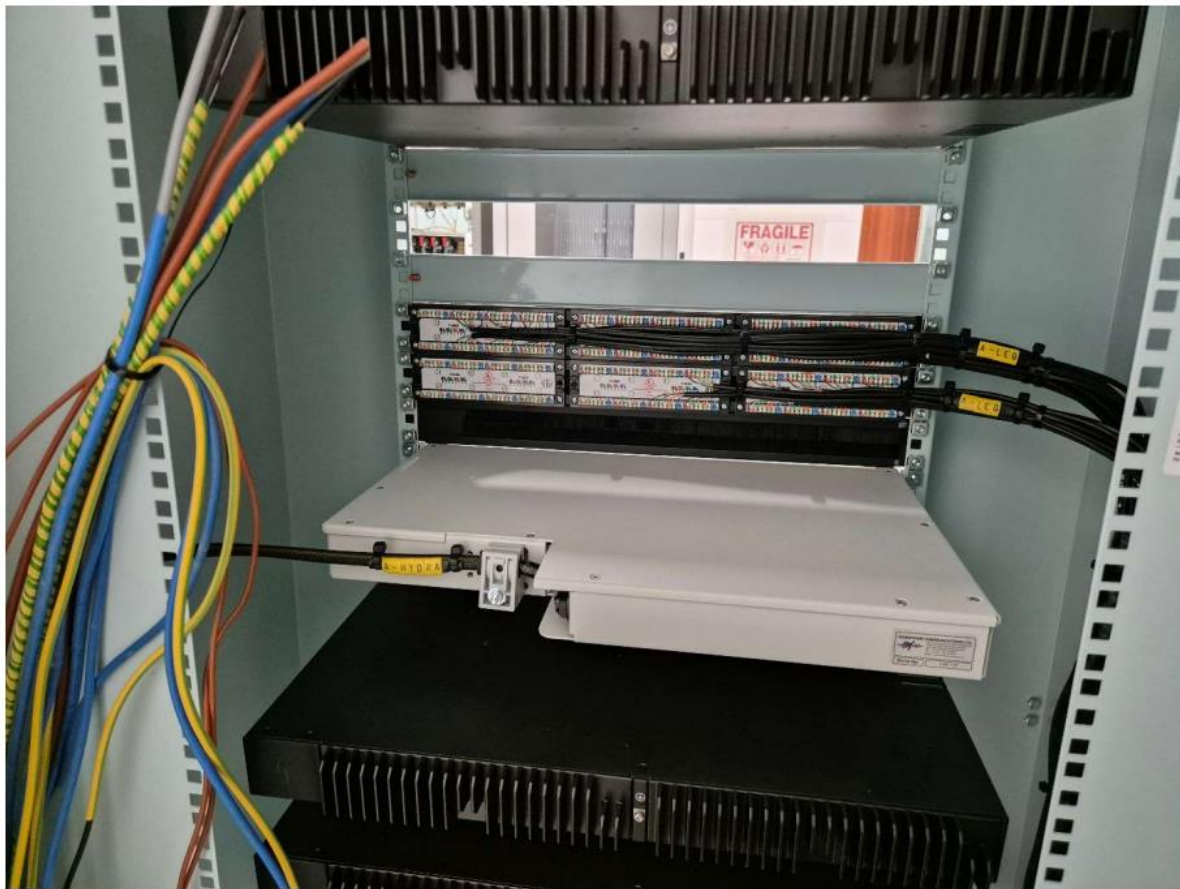
Figure 19: Example Wiring in Rear of a Grid Constellation Cubicle
