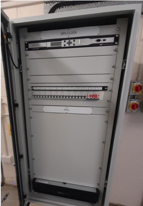
Figure 104: DER-4 PV – Constellation / RTU Cubicle
