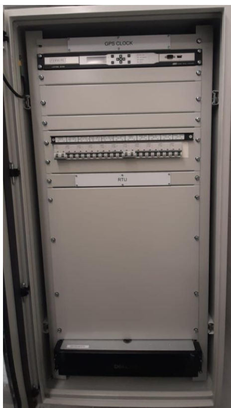
Figure 99: DER-5 – Constellation / RTU Cubicle
