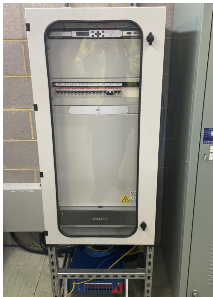
Figure 82: DER-1 Generation – Constellation / RTU Cubicle
