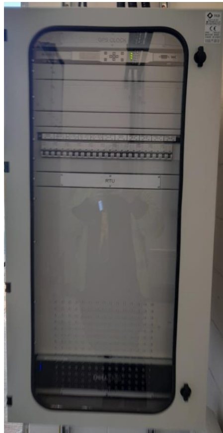
Figure 93: DER-2 – Constellation / RTU Cubicle
