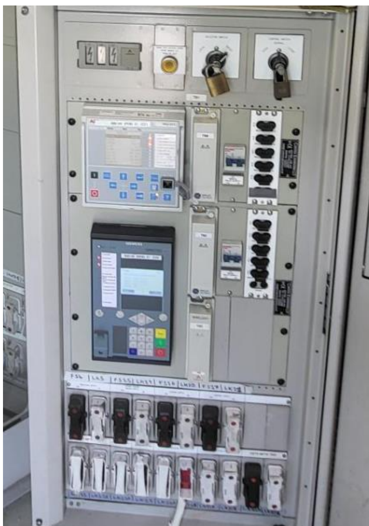
Figure 80: DER-1 Generation – Protection Panel
