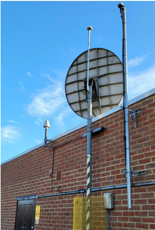
Figure 76: Maidstone Grid – GPS Antenna
