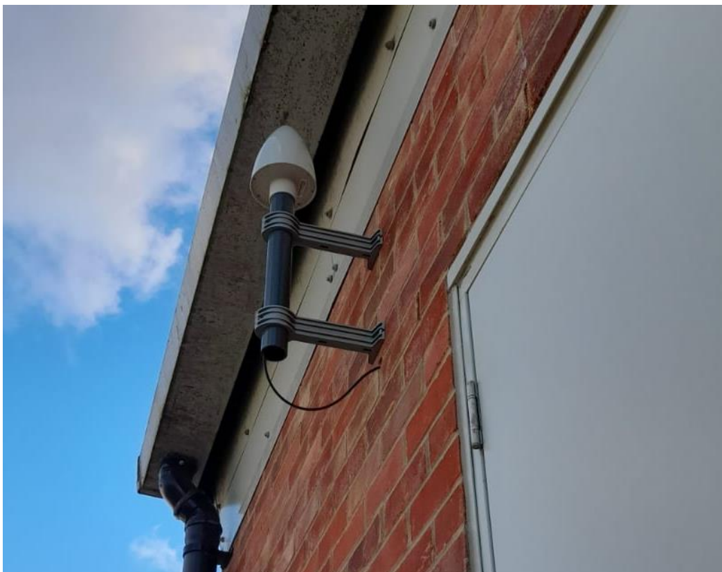
Figure 94: DER-2 – GPS Antenna
