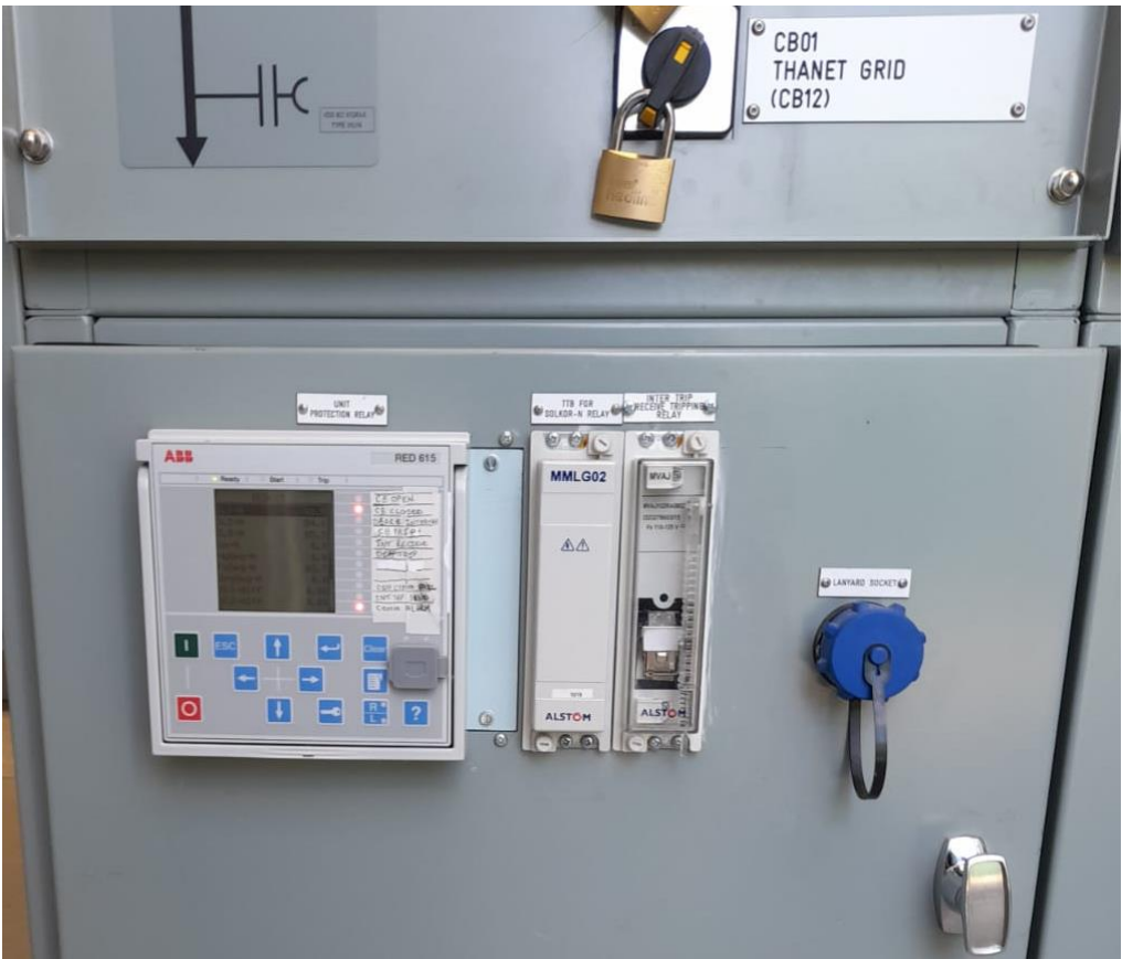
Figure 92: DER-2 – Typical Protection Panel
