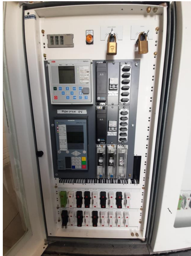
Figure 97: DER-5 – Protection Panel
