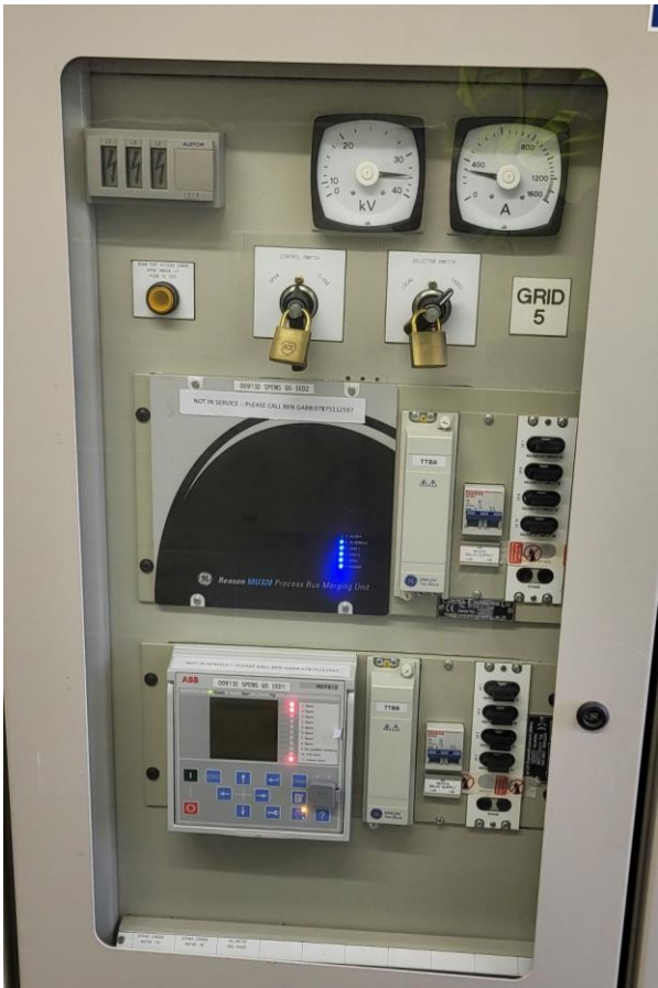
Figure 75: Maidstone Grid – Protection Panel Example
