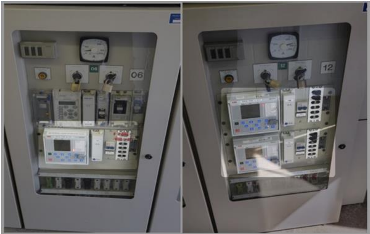
Figure 8: Examples of Maidstone Grid Switchgear Panels Containing Newly Installed Constellation Equipment
