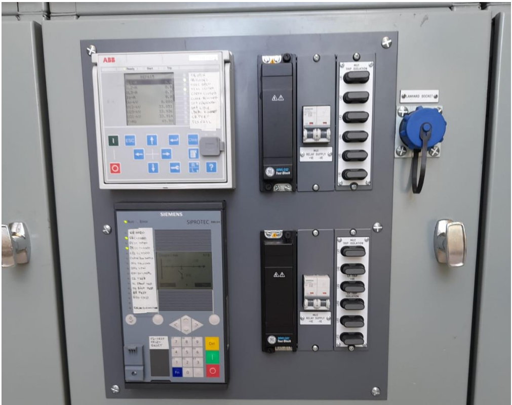
Figure 91: DER-2 – Typical Protection Panels (With Redundant Protection)
