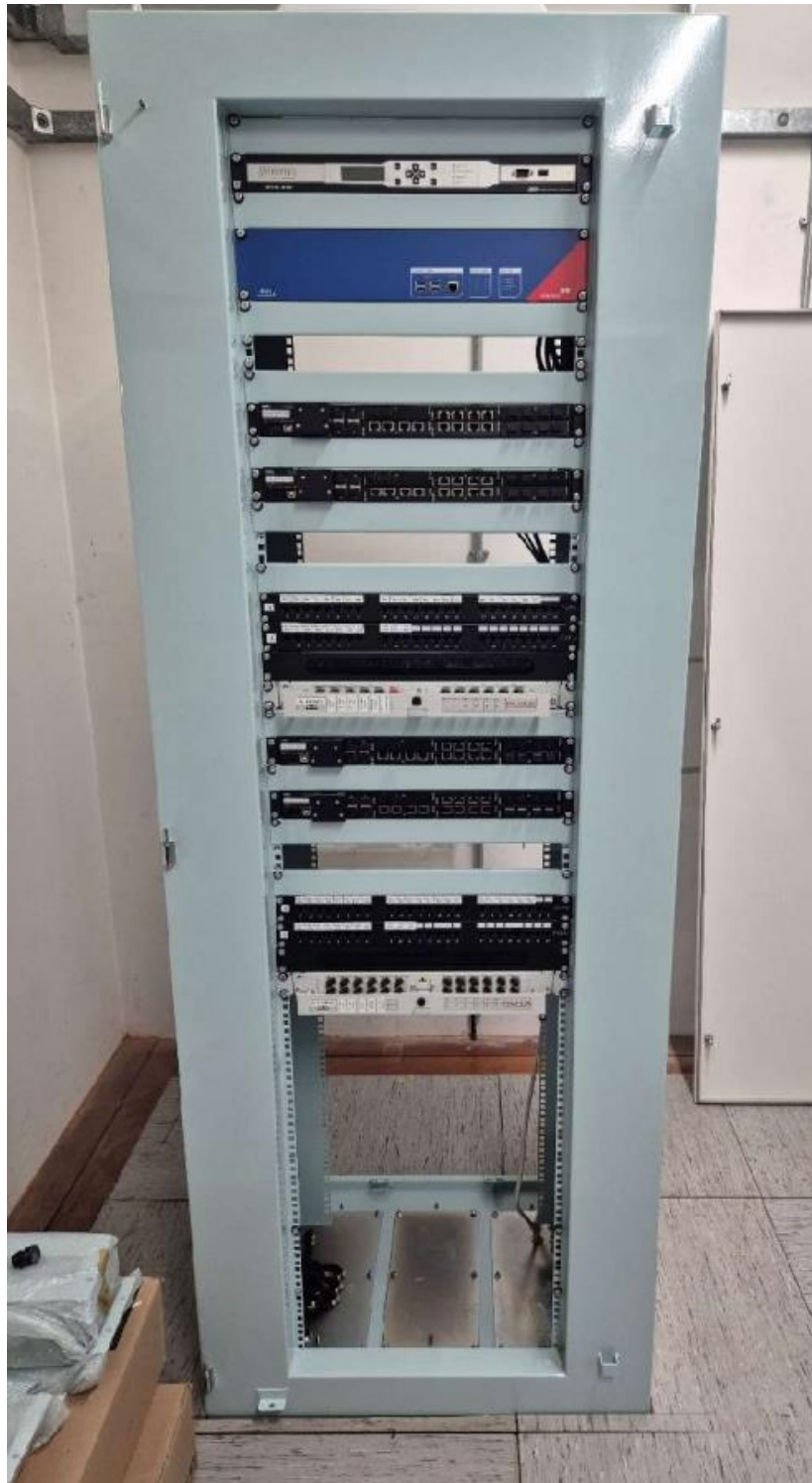
Figure 16: Grid Constellation Cubicle Undergoing Installation
