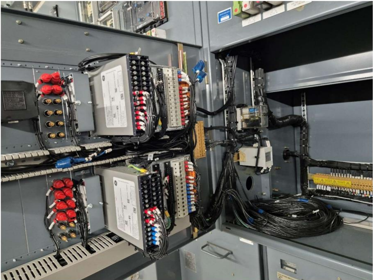
Figure 11: Example of Wiring the New Constellation IED Equipment in the Switchgear Panel
