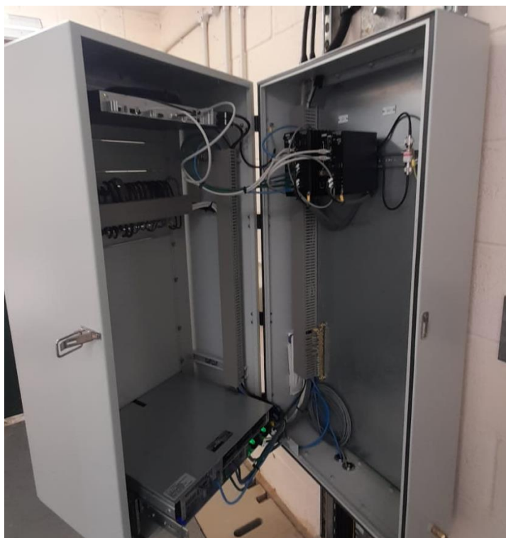
Figure 105: DER-4 PV – Constellation / RTU Cubicle (Interior)
