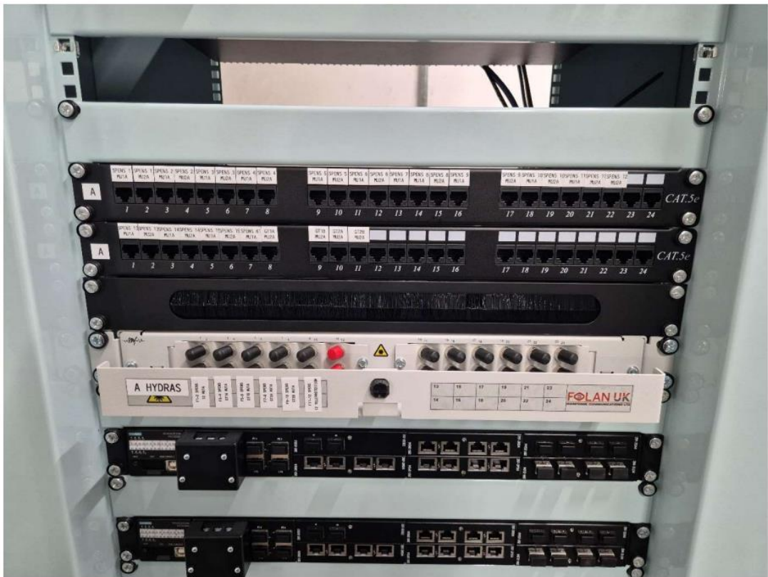
Figure 17: Close-Up Front View of a Grid Constellation Cubicle
