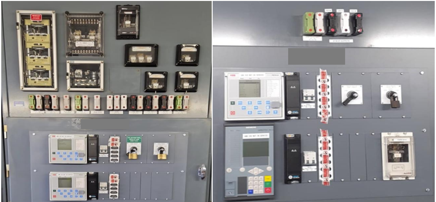
Figure 2-1 - New protection devices deployed in Thanet Grid
