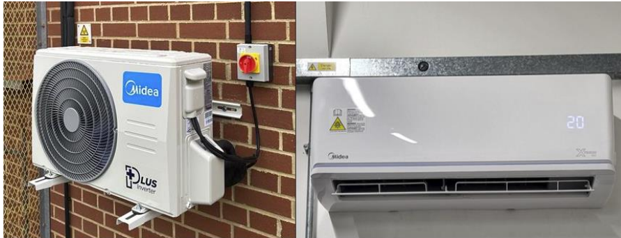
Figure 2-2: Air conditioning installed at grid site.
