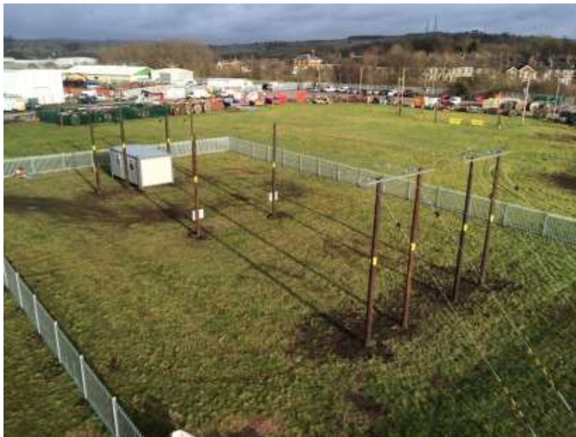
Figure 1 WPD Test Rig site
