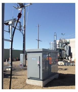
Figure 17 - SSFCL installed in Australia
