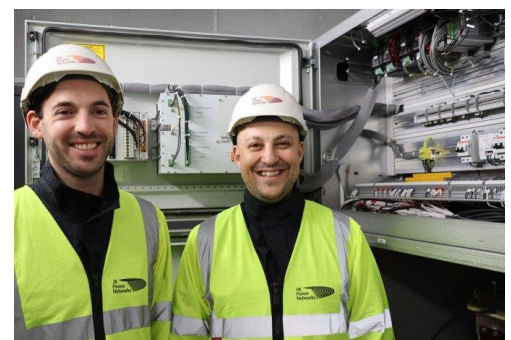
Figure 15: FLCB installation in Glaucus Street site
