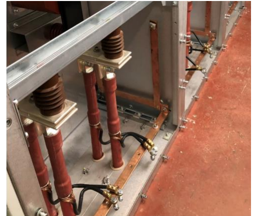
Figure 5: Completed HV cable terminations to the FLCB
