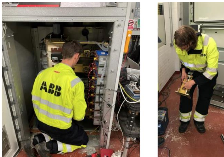
Figure 10: Site Inspection and Maintenance (left) and the mechanical switch replacement (right)
