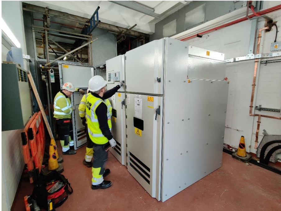
Figure 1 FLCB positioned into place and installation
