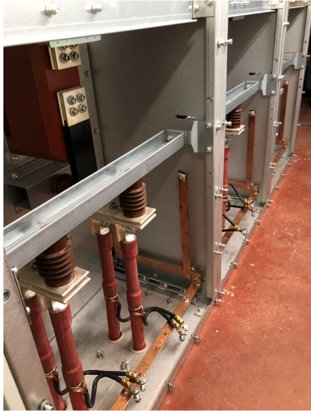
Figure 8 Completed HV cable terminations to the FLCB
