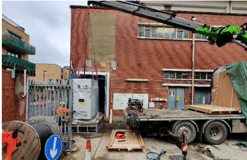
Figure 27 One panel of the FLCB being offloaded from the transportation vehicle
