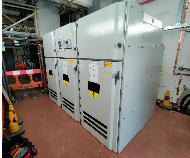
Figure 29 FLCB installed in final position and reassembled
