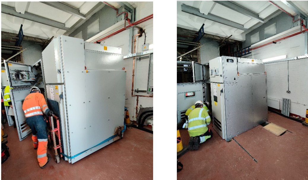
Figure 28 FLCB panels being shifted into place
