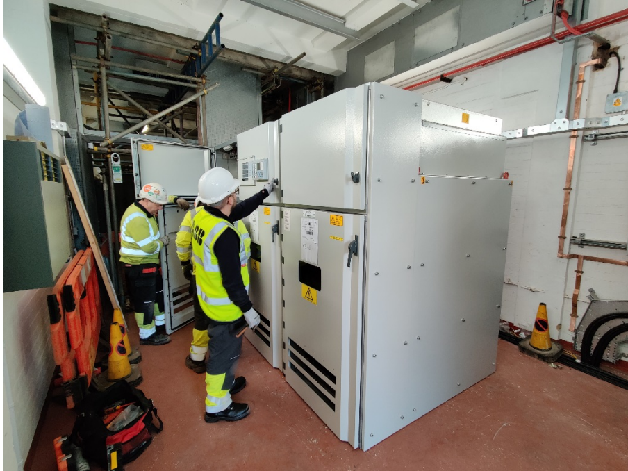
Figure 1 FLCB installation in progress
