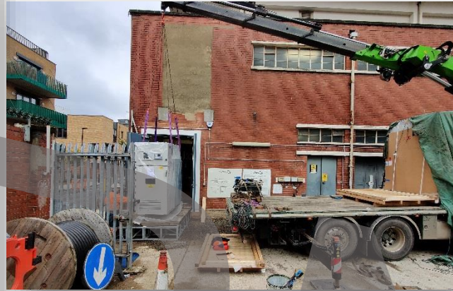
Delivery of FLCB to site
