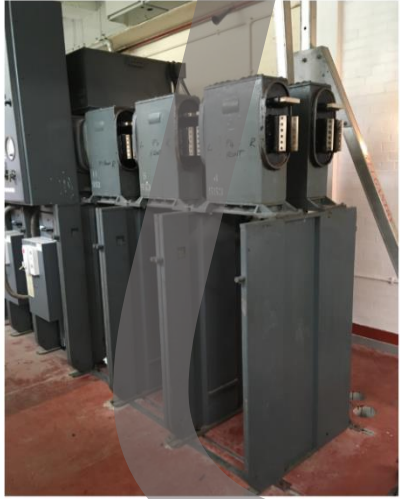
Extension of existing busbar to include 2x feeder panels
