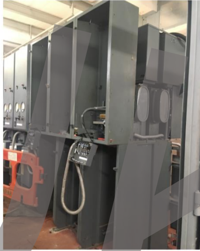
Extension of existing busbar to include 2x feeder panels
