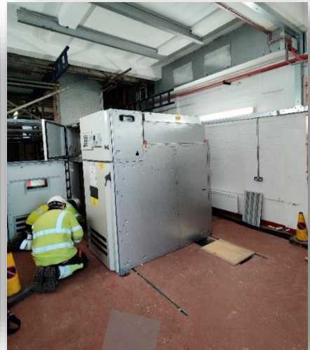
Installation of FLCB
