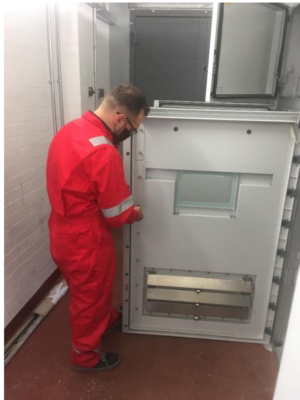
Figure 1 FLCB HV door interlock being repaired
