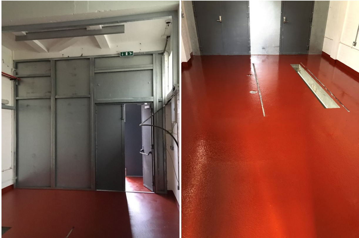
Figure 7 Finished preparation of the room ready for FLCB installation
