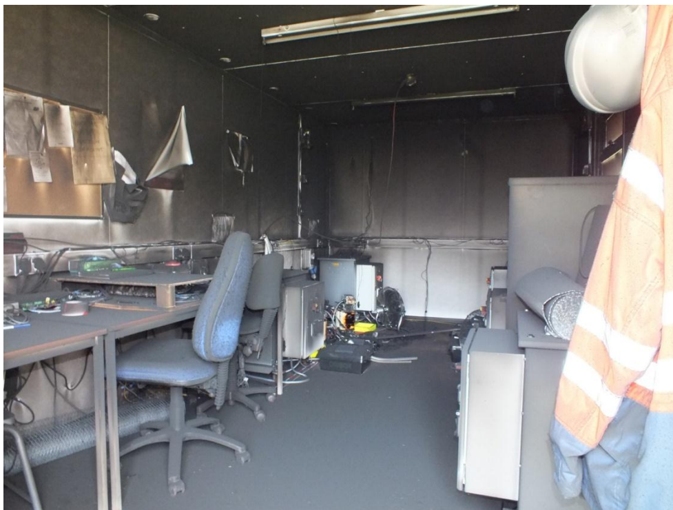
Figure 1 General view inside Porta-cabin 7 th June 2016
