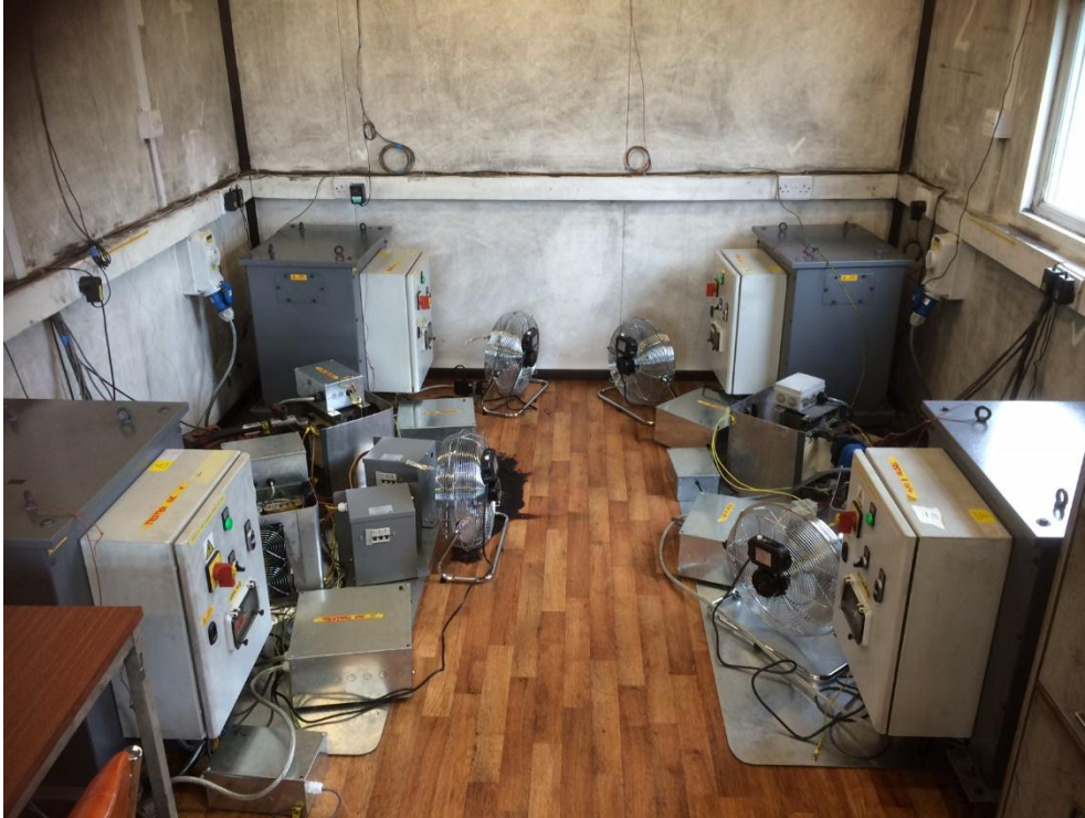
Figure 3 Porta-cabin following reparation work 5 th August 2016
